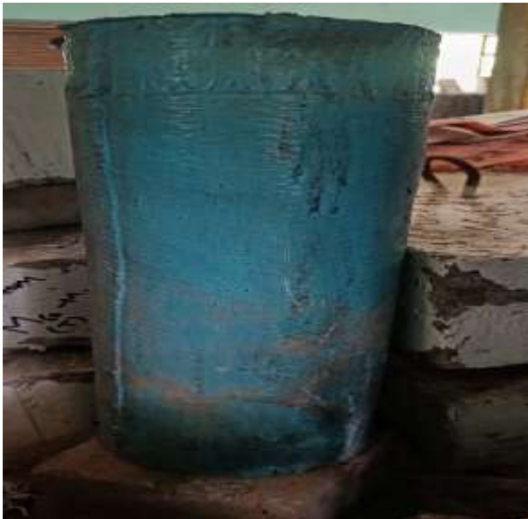
Fig 7 Failure of Strengthend column (debonding stress )
