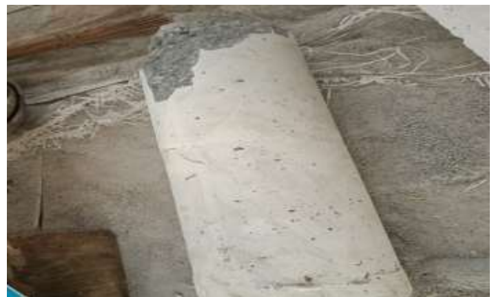
Fig 6 Failure of concrete column
